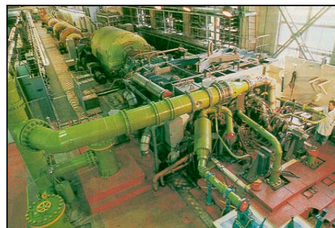
Figure 11. NPO Energomash Water Flow Test Facility
