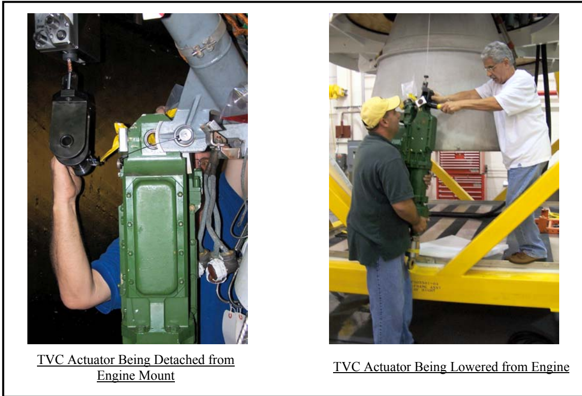
Figure III-5 Removal of RD-180 TVC Actuator Conducted During Trial Removal
